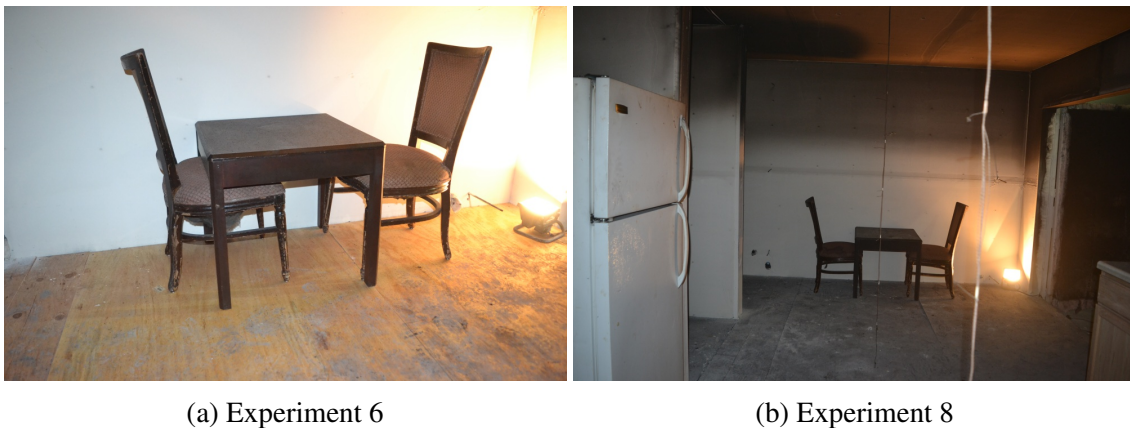
Figure 6.25: Post-suppression comparison of kitchen dining area opposite area of origin with closed door.
